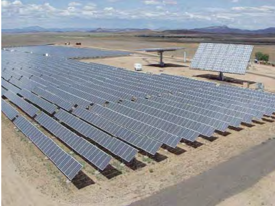
Figure 5.2.1. Arizona Public Service's Prescott Airport Solar System Showing a Tracking Flat-Plate, Nonconcentrating PV System. In the background are concentrating PV systems. (Source: Herb Hayden, Arizona Public Service)
