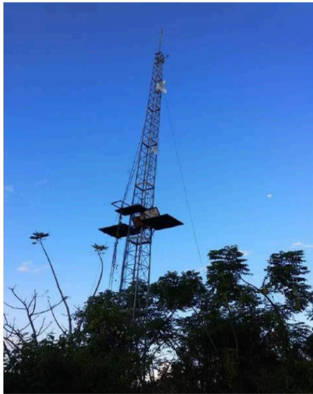
Figure 7: Wireless network tower on Bunaken Island.
